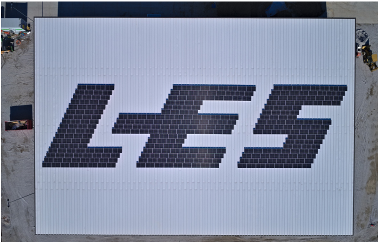
Aerial views of the rooftop solar array of 142 kW on LES' Reel & Transformer building. With the additional 76 kW of solar on the LES carport, LES has a total of 218 kW of solar at the Operations Center.
